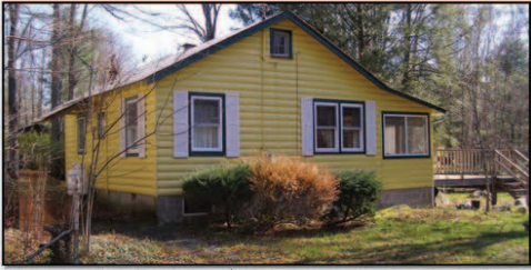
Storybook Charmer $174,900 Charming interior with designer's loft. Huge private deck overlooks a splendid yard at the end of a dead end road. Smallwood Lake community offers lake access with beach, dock and sports court. Enclosed porch, fireplace, and skylights. Really Sweet! #18338
