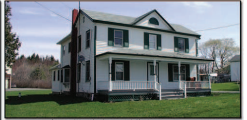
Moments from "Bethel Woods" $849,900 Frontage on RT-17B! Zoned Gateway Commercial, with gorgeous 19± beautiful acres. Excellent exposure for numerous commercial opportunities. Renovated 5BR farmhouse, a 2-bay garage with income potential and guest quarters, shed, paved parking, in a FABULOUS location!! #19128
